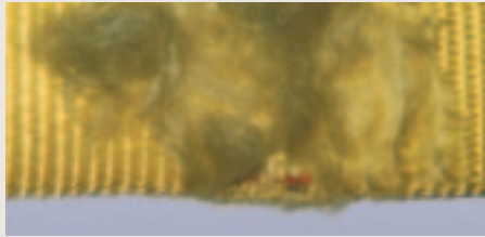
Excessive abrasive wear
